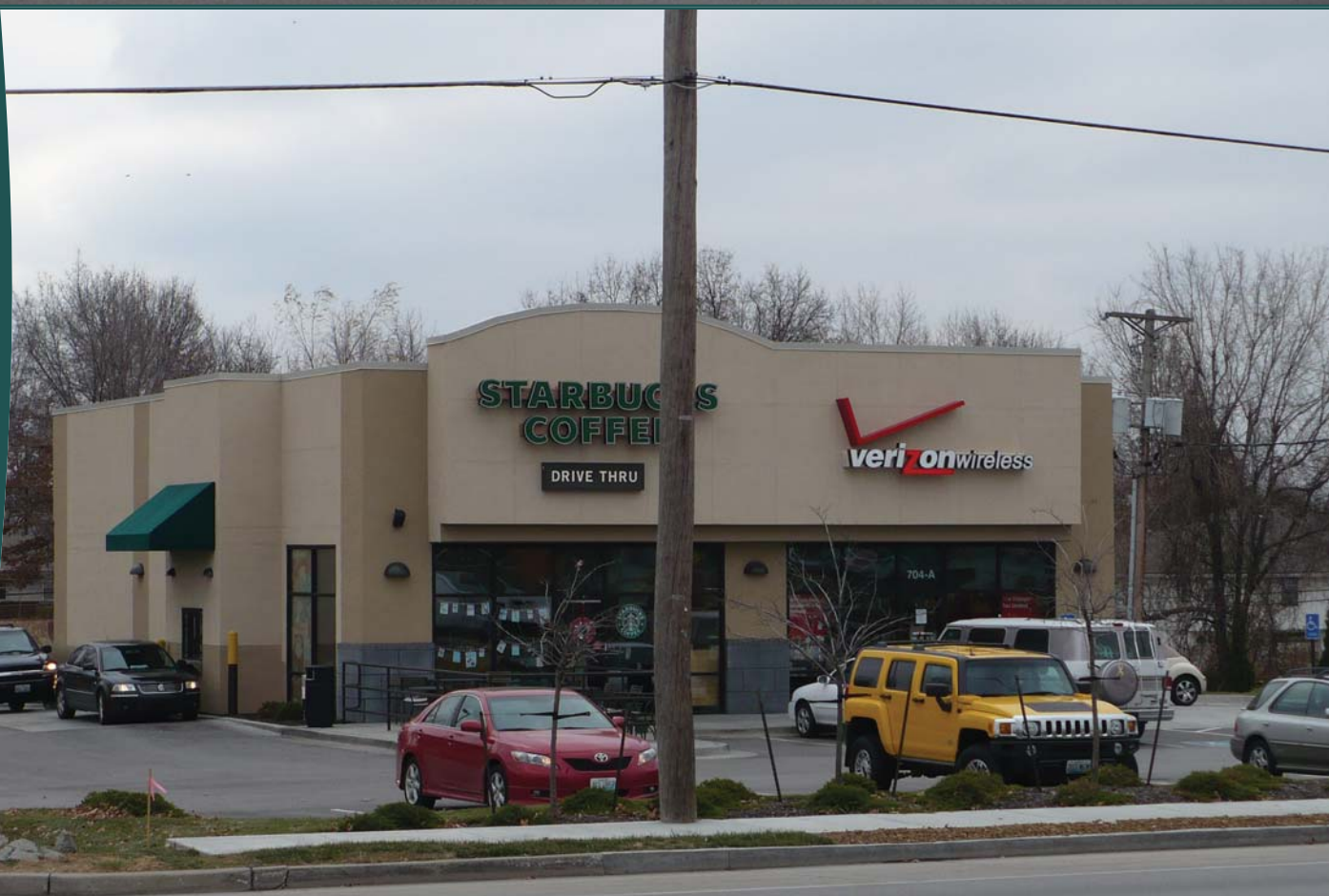
Newly built Retail Property: 100 yards South of Subject Property
